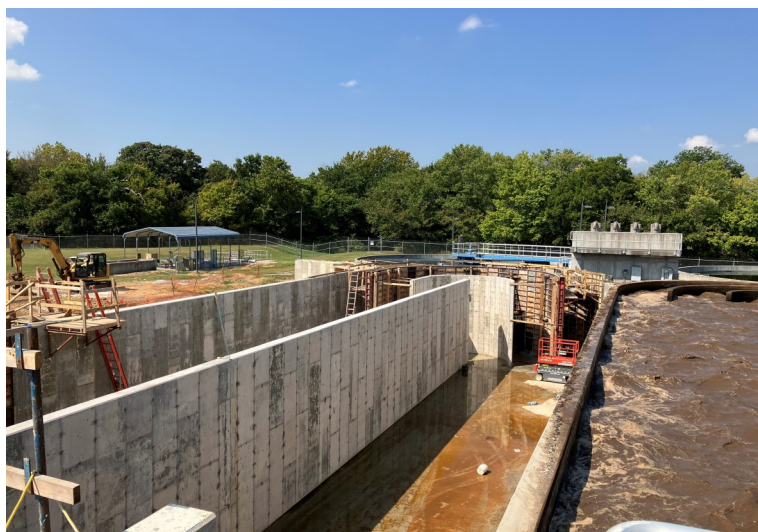
Bottom: Bio Unit #3 is almost ready to fill with water for testing.
